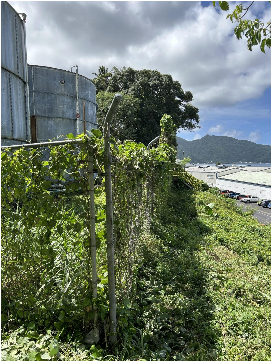
Figure 3: Picture of the Front View of the Two Existing STP Tanks, Perimeter Fence, Roadway Below and the StarKist Plant across the Street
