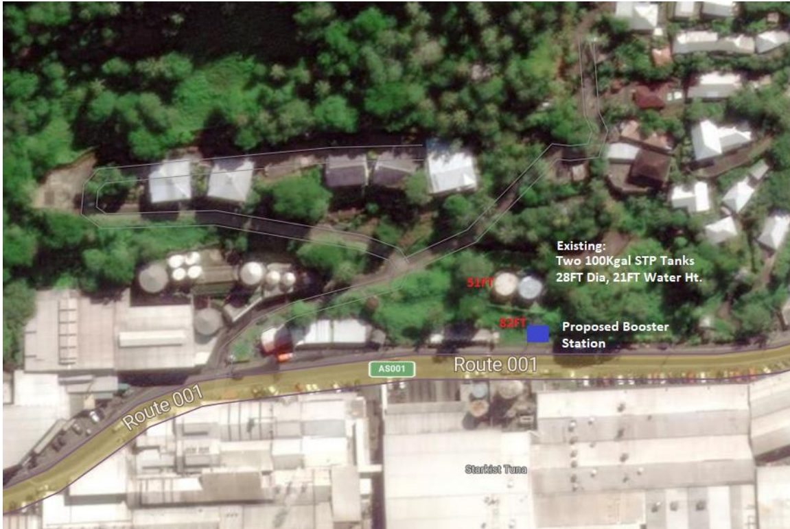
Figure 1: Aerial View of Existing Site
